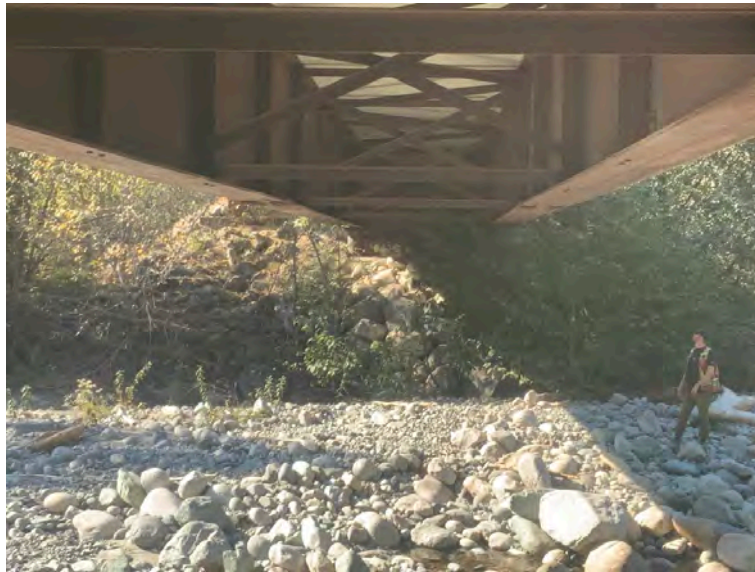
Right Bank Abutment when facing downstream
