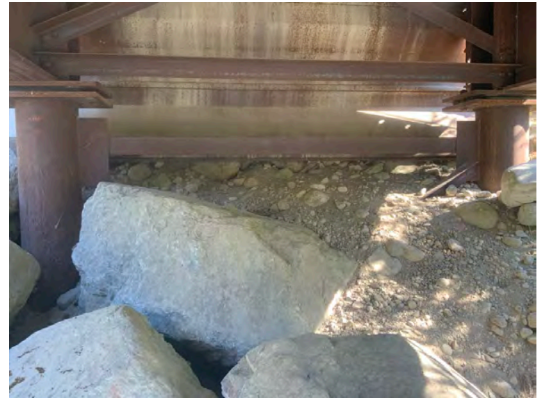
Left Bank Abutment when facing downstream
