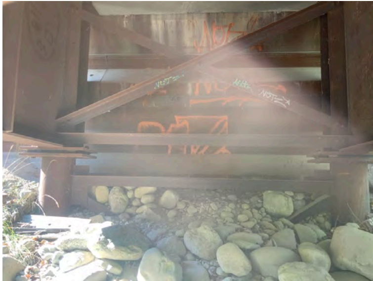
Right Bank Abutment when facing downstream
