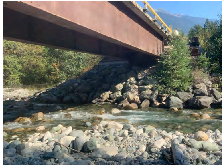
Left Bank Abutment when facing downstream
