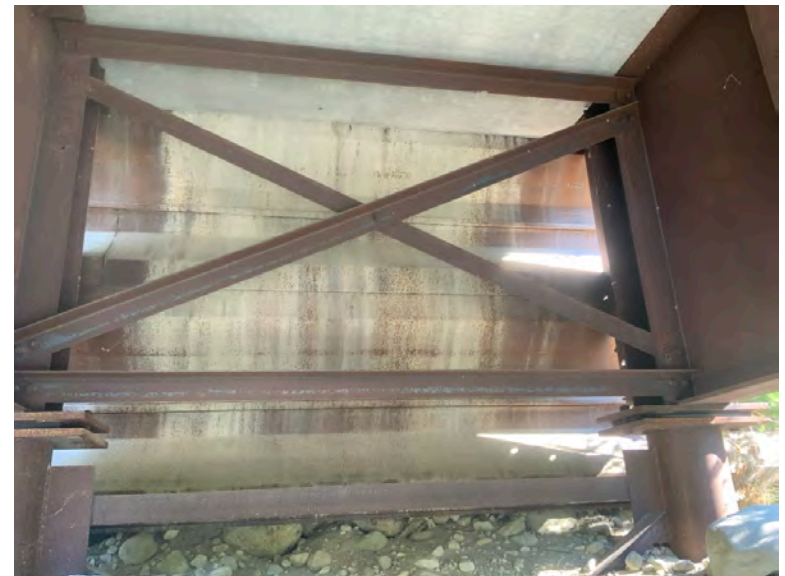
Left Bank Abutment when facing downstream
