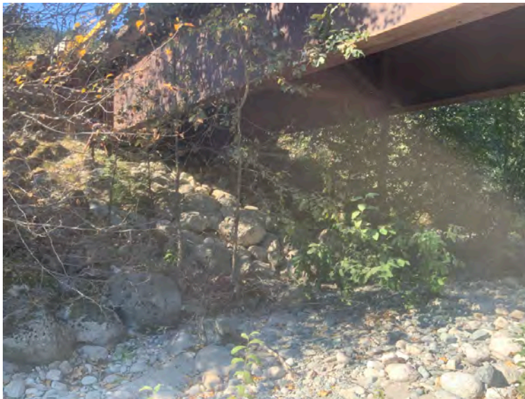
Right Bank Abutment when facing downstream
